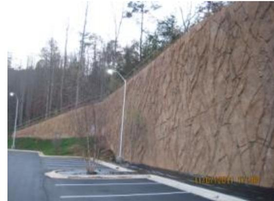
Deep cuts were made into the hillside at the rear of the structure. The excavation is supported by two permanent soils nail walls which were terraced to provide the required excavation depth. Wall heights are as much as 35 feet. Total face area soil nailed was about 33,516 ft<sup>2</sup>.
